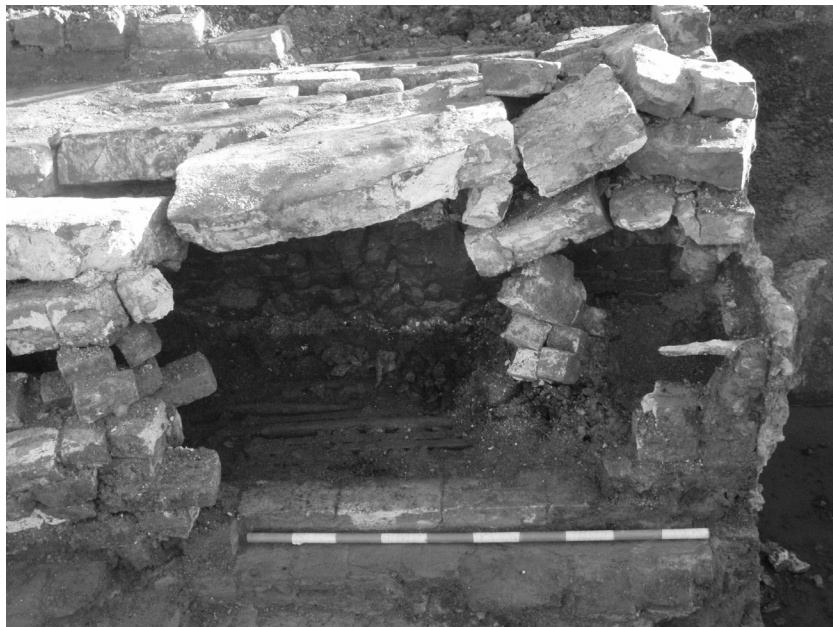
Figure 11. Detail of the No. 6 furnace showing slagging on bricks and the remains of coke along back of furnace. The cheek plate (right) has burnt away.
