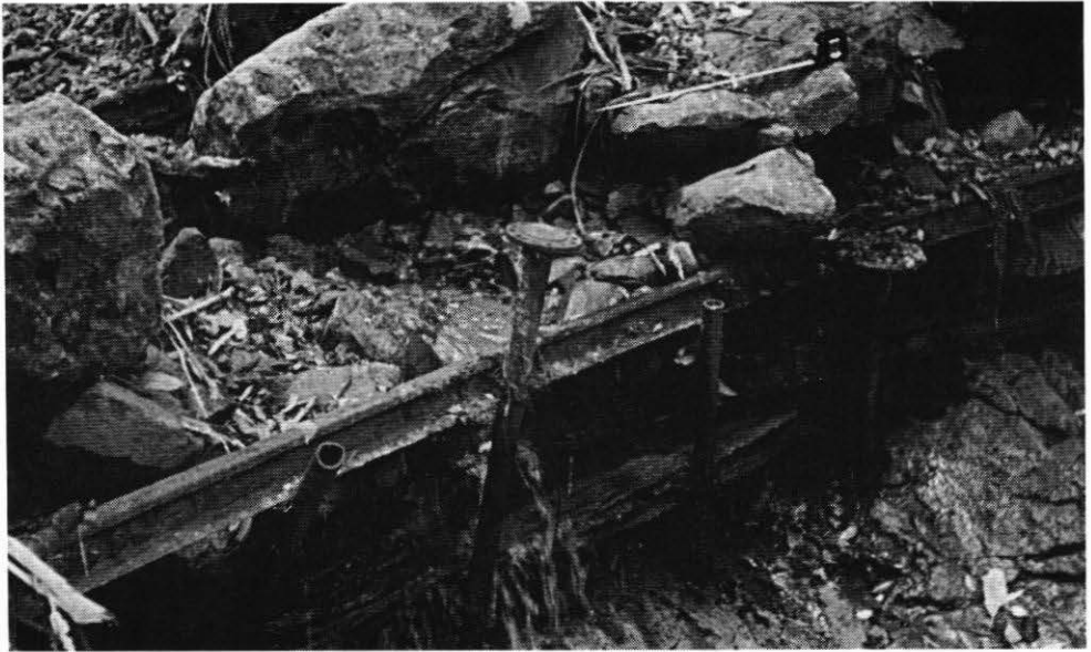
Figure 4. Stanchions placed across Diamond Creek crossing.
