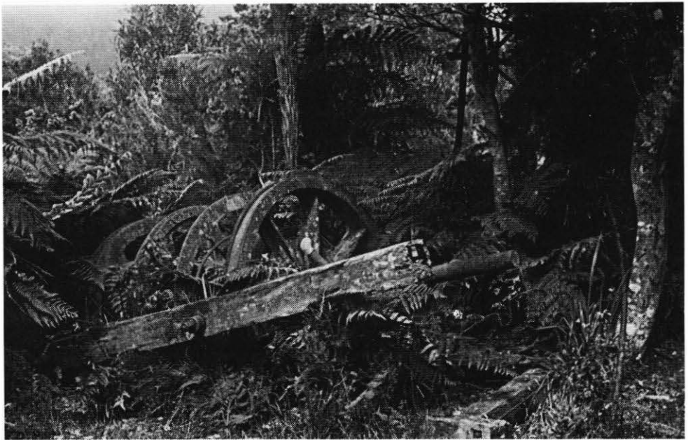
Figure 5. Butler's Incline brake and winding gear.
