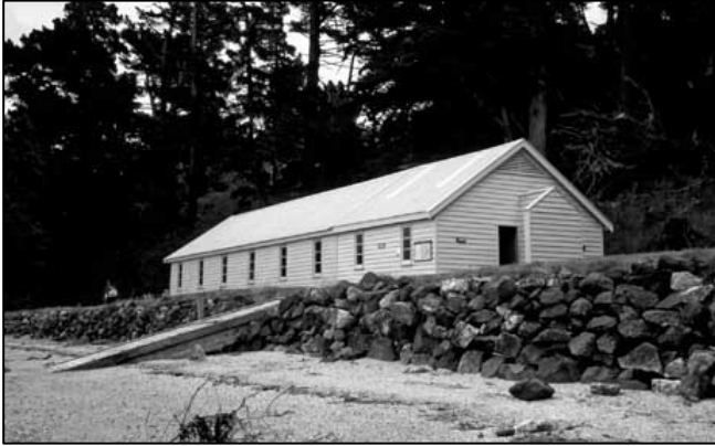
Figure 4. Single Men's Quarantine Barracks Quail Island (Gavin McLean https://nzhistory.govt.nz/media/photo/quail-island ).
