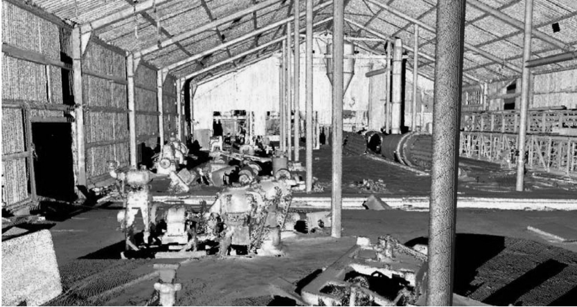
Figure 4. Interior scan of the guano factory, Husvik.
