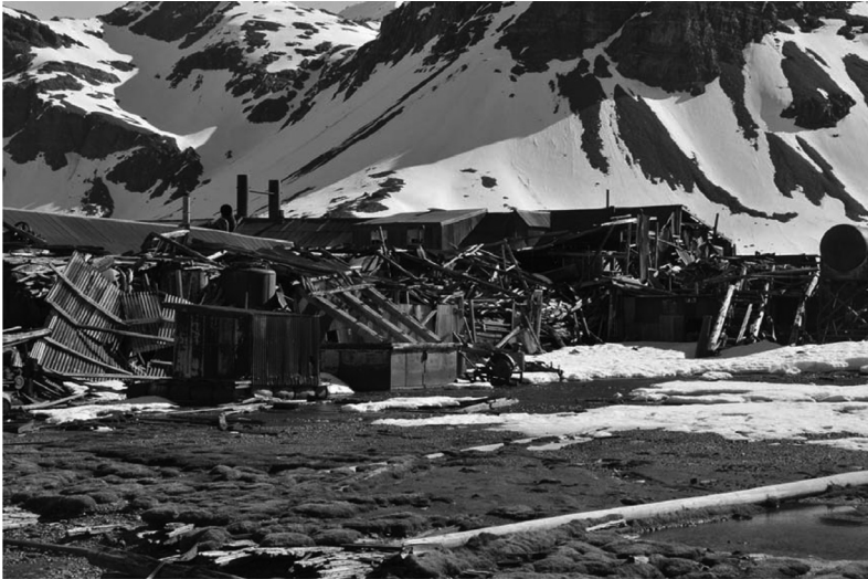
Figure 3. The flensing plant (foreground) and partially collapsed production plant, Husvik.
