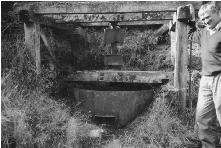
Figure 3. Turbine installation at Bella Reef, Waipori.
